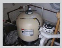
Pool was not winterized properly resulting in a cracked filter tank and plumbing lines.
